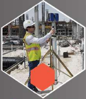
Construction Process Monitoring
